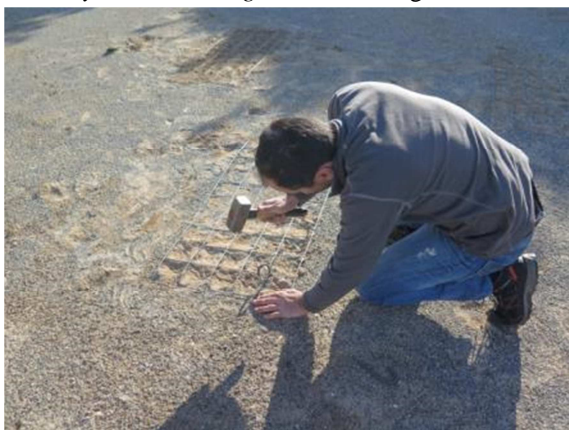
Metal grid stabilization & Planting of seedlings within fenced area
